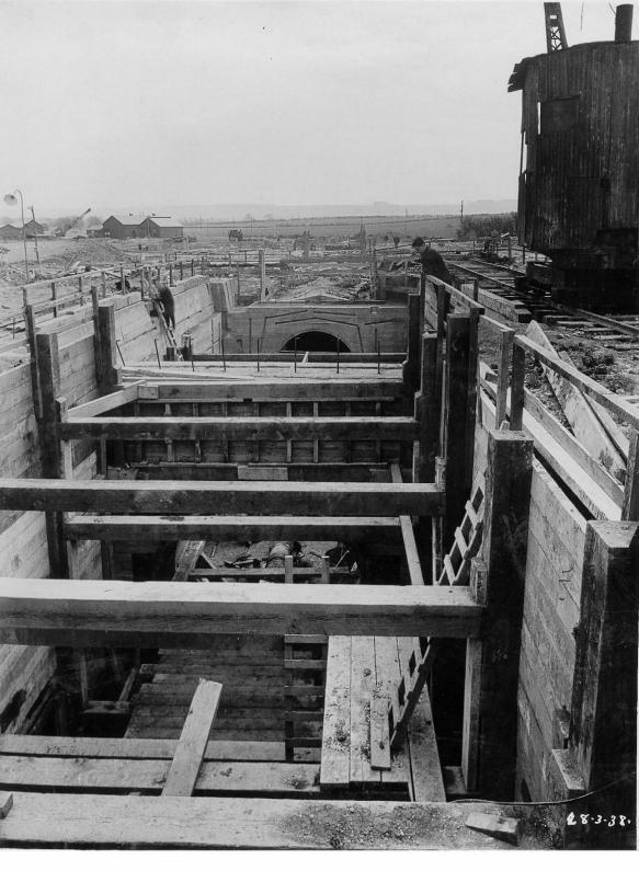
1. Construction of concrete tunnel for position of overflow. 2. General view. looking toward Mutland. 31 Different stages, looking towards Eutland. Construction of concrete 41 diaphram, also view of old stream for diversion. 6. Early construction of diversion tunnel looking towards Rutland. Heap of top soil in little distance towards right.
